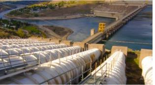
Steamboat Rock State Park is on Banks Lake, and that lake was created by filling the Grand Coulee with Columbia River water. Electricity generated at the dam is used to pump water up to the coulee where the water is mainly used for irrigation. Some water can also be released back to the turbines at the dam to make electricity at times of peak demand.
